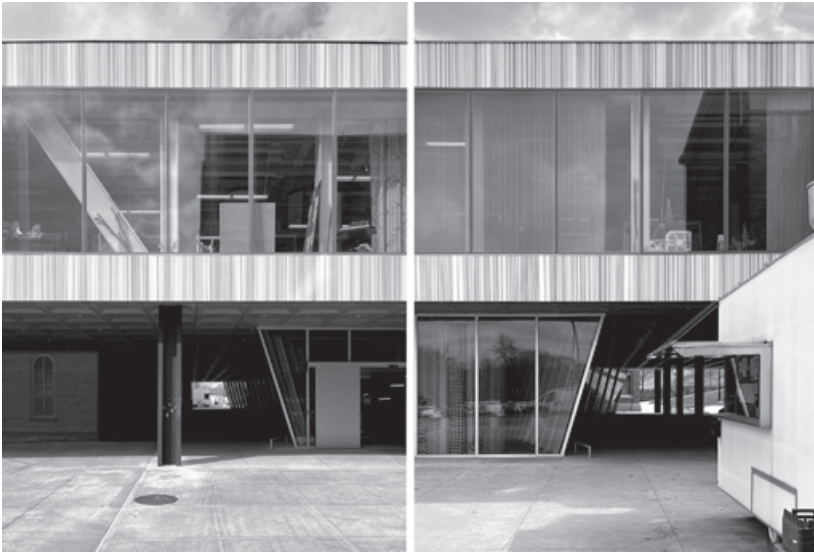
Figure 4.4. Milstein's arcade, viewed from the Milstein plaza ( right ) and from outside Rand Hall ( left ), remains dark and uninviting, even with soffit lights and integral curtain wall mullion fixtures turned on.
