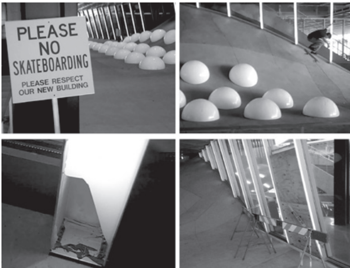
Figure 6.10. Skateboarders are warned away from Milstein Hall's dome ( top left ) but show up anyway ( top right ); lighting fixtures and glazing panels have been damaged ( bottom left and right ), possibly from collisions with skateboards.
