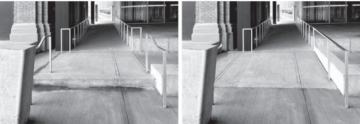
Figure 6.18. The single step at the end of a ramp leading from the Main entrance (exit) from Milstein Hall to University Avenue represents a noncompliant elevation change ( left , as-built image); simply extending the ramp to the University Avenue sidewalk would have eliminated that problem ( right , photoshopped image).
