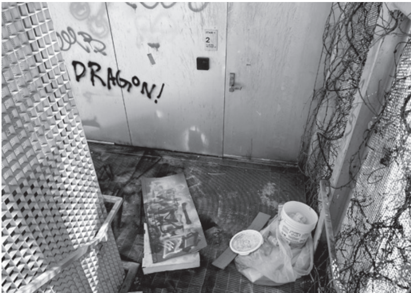
Figure 7.14. The exterior stairway on the west side of Milstein Hall has been appropriated as a de facto spray paint booth, solid waste disposal site, and smoking room, but certainly cannot function as “boundless studio space.”
