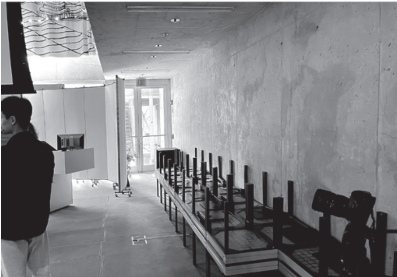
Figure 3.4. Position of an exit door in Milstein Hall's auditorium makes it difficult to productively use the space immediately adjacent to the side wall for either seats or required exit access. Peter Eisenman inaugurates the "Peter Eisenman Lecture Series" ( top ) on April 26, 2023, with a story about Colin Rowe and a certain Palladian villa projected on the screen, seemingly oblivious to the blocked exit door immediately to his left; the same blocked exit door is viewed from ground level ( bottom ).
