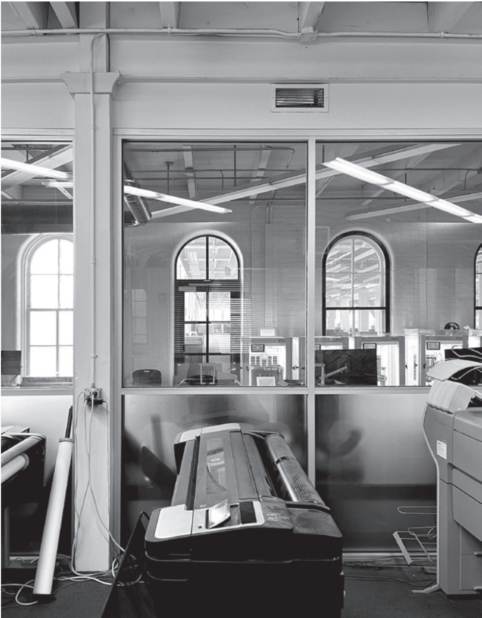
Figure 24.2. Sibley Hall's digital fabrication lab, immediately adjacent to Milstein Hall (visible through the fire barrier windows), has no fresh air supply—except for what gets in the room through transfer grilles visible above the glazed wall—in spite of containing 3-D printers, some of which use material that is both toxic and carcinogenic.
