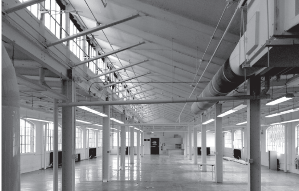
Figure 15.7. Rand Hall’s non-fireproofed steel frame in 2017, before it was converted into the Mui Ho Fine Arts Library.
