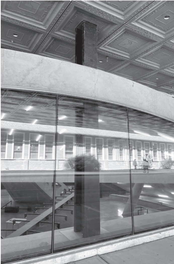
Figure 9.12. Exterior column No. 4 penetrates both the second-floor soffit above and the Crit Room space below.
