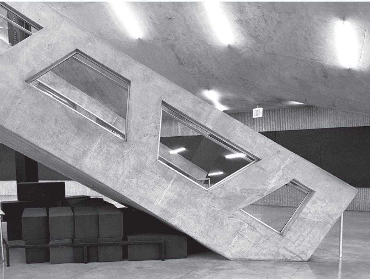
Figure 3.3. Highly combustible foamed plastic display stands are stored under the Crit Room exit stairway.
