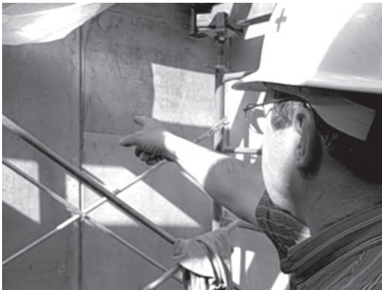
Figure 11.22. The contractor's field superintendent explains the mottling of concrete surfaces in Milstein Hall's Crit Room.
