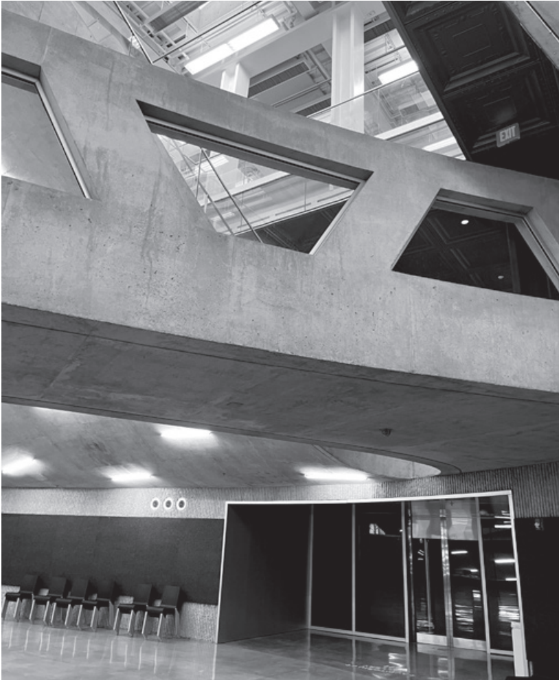
Figure 4.16. Lobby-Crit Room-studio interpenetration: The spatial excitement of interconnected spaces at three levels results in acoustical conflicts between circulation (over the trussed bridge at the entry level), second-floor studio spaces, and the Crit Room below.
