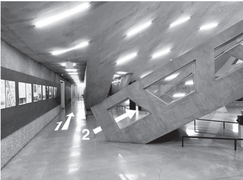
Figure 16.3. The Crit Room only has two exit access doors or openings: an exit access opening (1) leading to an exit near the gallery; and an exit access stair (2) leading to second exit at the main entry level within the Crit Room.
