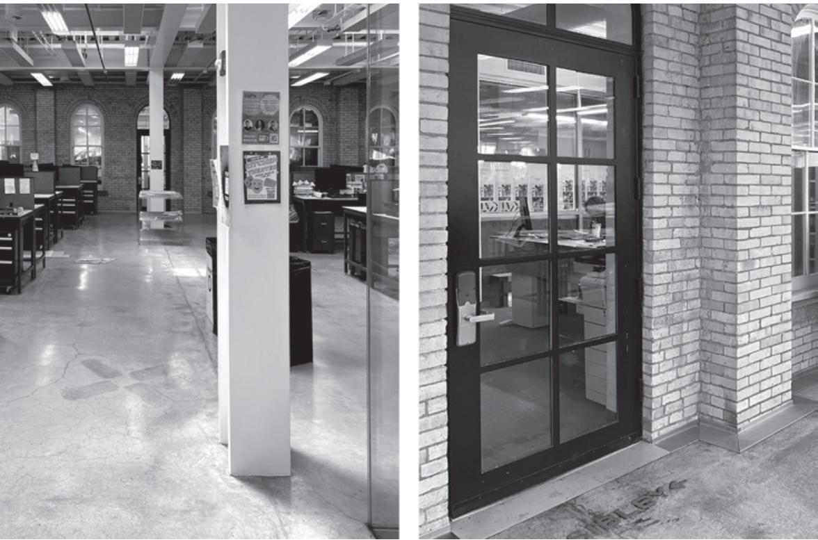
Figure 5.5. One of the four doors linking Milstein and Sibley Halls provides access to an IT support room, visible behind the glass door ( right ); in Milstein Hall, the circulation aisle to this door is bisected by a row of steel columns ( left ).
