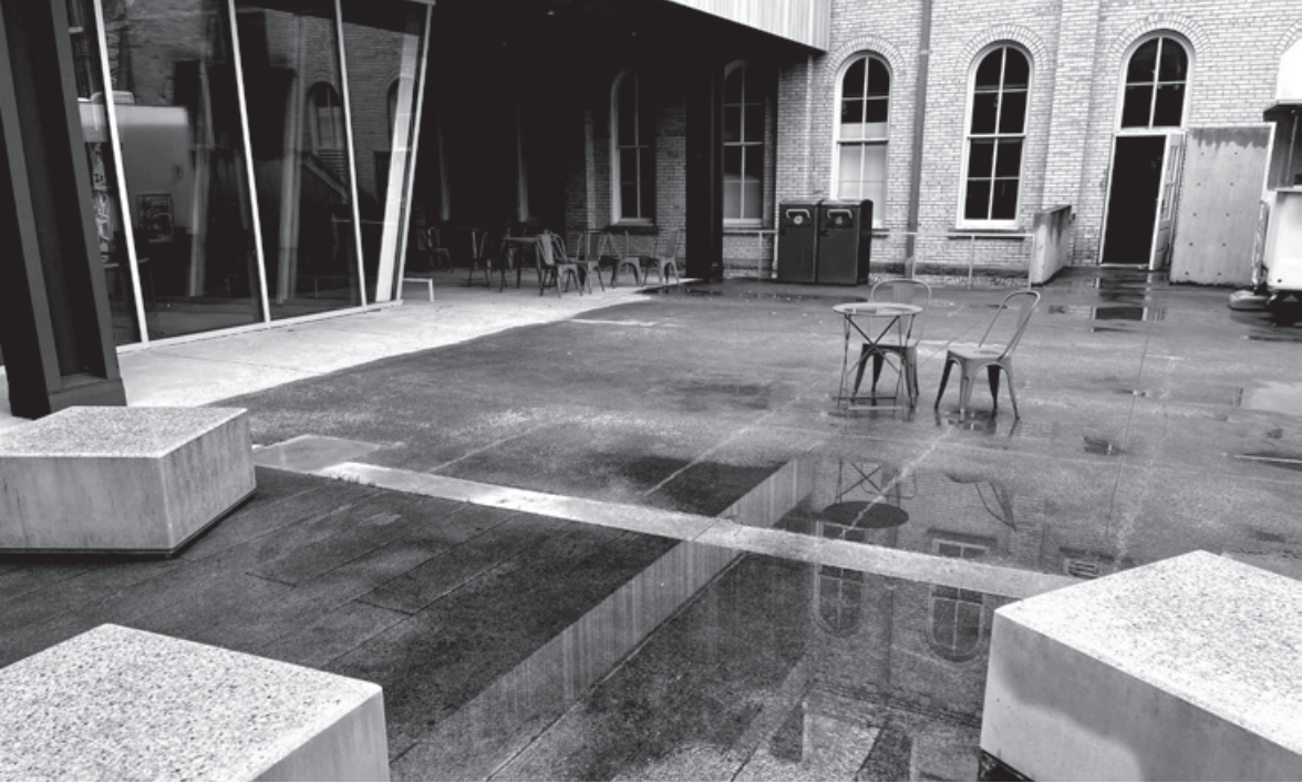
Figure 10.17. Puddles still form, and remain, on the Milstein Hall plaza because the slope caused by the slab's unintended deflection does not create a consistent low point that aligns with the position of the linear drain that was added later, visible in the middle of the image.
