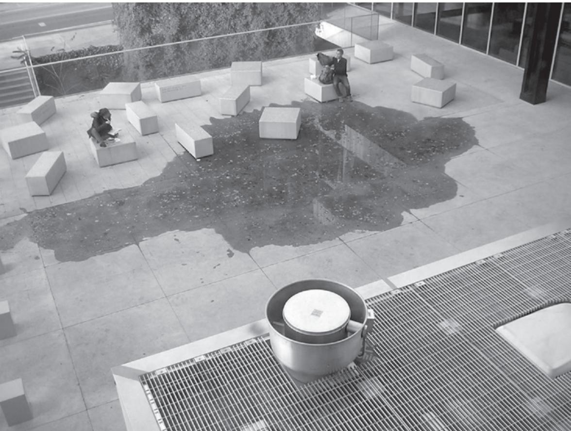
Figure 10.12. Water would pool at the center of Milstein Hall's plaza long after any rain had stopped, for two reasons: first there was no drain; and second, the slab deflected so that rainwater tended to move to the center of the concrete deck's span.
