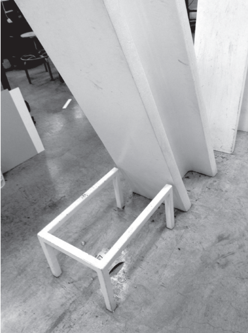
Figure 6.20. Typical cane-detection guard at inclined (protruding) structural element in Milstein Hall.
