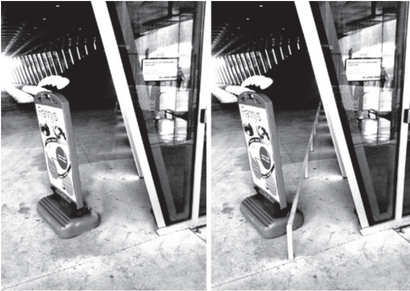
Figure 6.23. Cane-detection guards were added to the sloping curtain wall in the arcade: before, simulated ( left ) and after ( right ).
