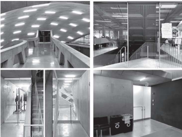
Figure 4.14. Glass doors provide no acoustic isolation for the auditorium. From top-left, clockwise: glass door from entry-level bridge; glass door from second-floor studios; glass doors into adjacent crit room; and glass door to corridor.
