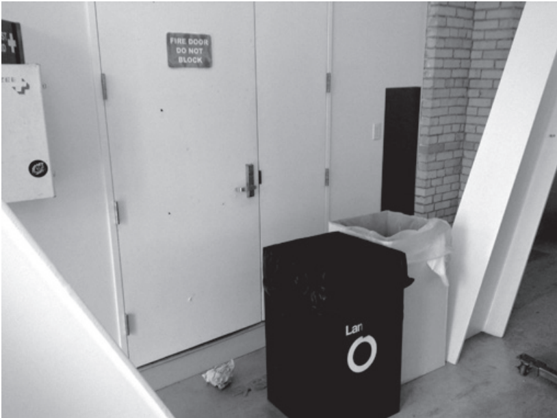
Figure 5.4. The fifth door connecting Milstein Hall and Sibley Hall was changed from a glass wall and door in Sibley Hall's eastern loadbearing wall—the opening was created at great expense to allow for this expanse of fire-rated glass—to an ordinary steel door with the adjacent space unceremoniously filled with fire-rated gypsum board. At the time of this writing, the door has been removed and the opening has been covered with fire-rated drywall.
