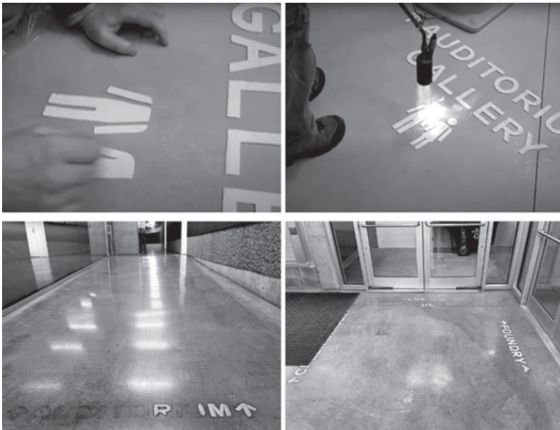
Figure 6.12. Milstein Hall’s signage system is assembled with individual letters and symbols that are placed on the concrete slab ( top-left ), torched onto the concrete surface ( top right ), and then left to be damaged or destroyed by foot traffic and cleaning protocols ( bottom left and right ).
